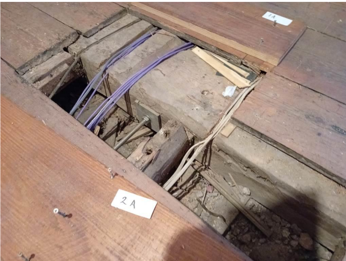
Photo 24: Merchants House: The oak carrier beams in the 1 st floor 'Parlour'
