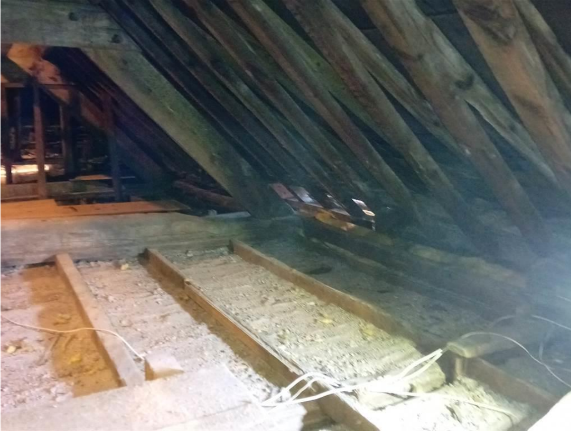
Photo 7: Merchants House: Typical view of the roofspace.
