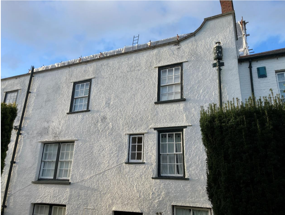
Photo 3: Side elevation of the merchant's house viewed from the enclosed courtyard.
