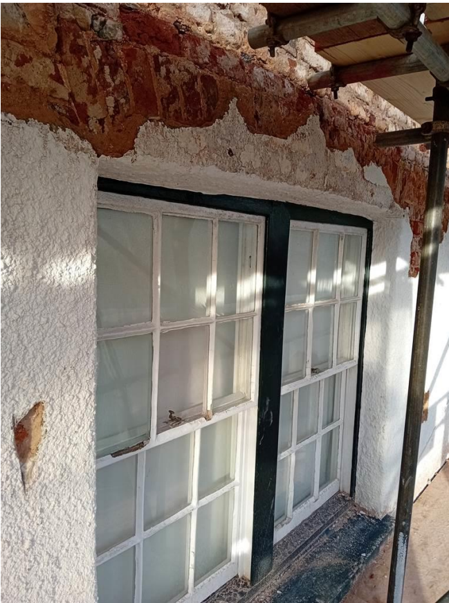
Photo 28: Merchants House: Typical brick arch to the original window openings
