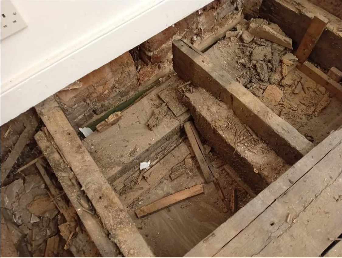
Photo 21: Merchants House: The floor joists in the 2 nd floor 'Records Store'
