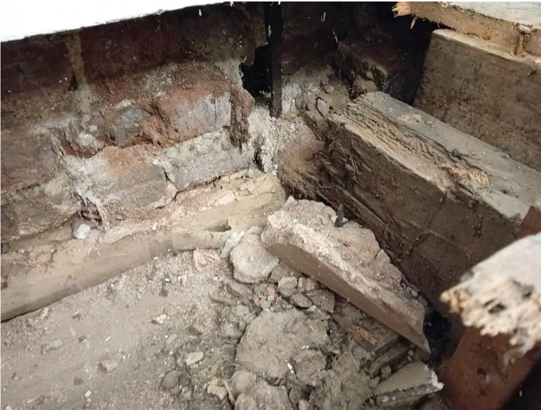
Photo 23: Merchants House: The floor joists in the 2 nd floor 'Records Room'
