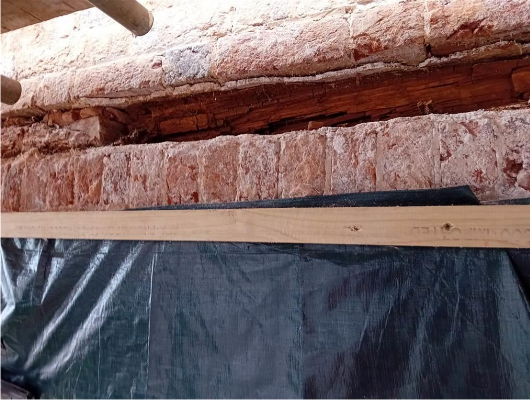
Photo 27: Merchants House: Wall plate no.1 built into the external walls.
