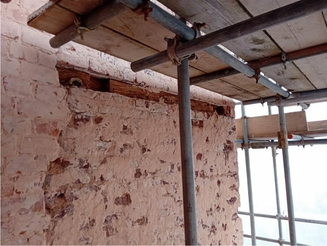
Photo 25: Merchants House: Wall plate no.3 built into the external walls.
