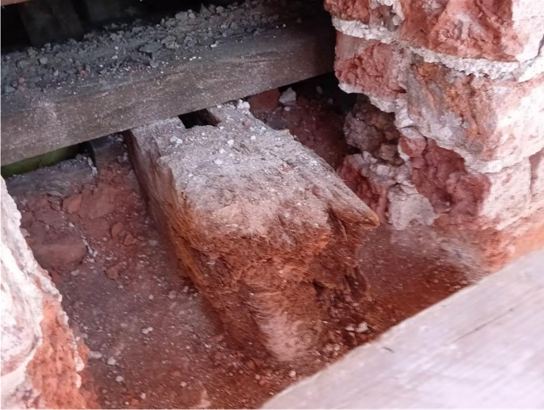
Photo 11: Merchants House: View of the bottom chord of a roof truss built into the external walls.
