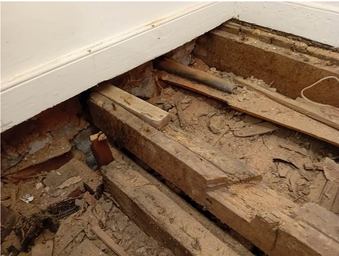
Photo 22: Merchants House: The floor joists in the 2 nd floor 'Records Store'
