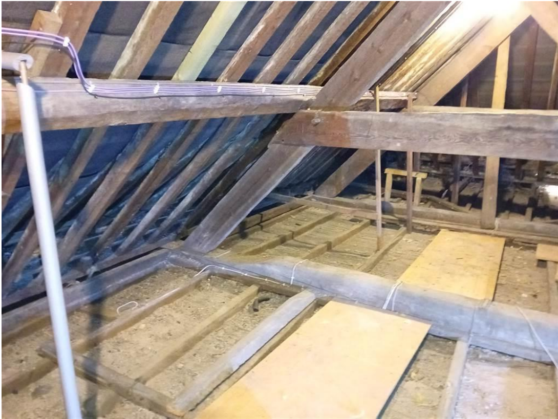
Photo 6: Merchants House: Typical view of the roofspace.
