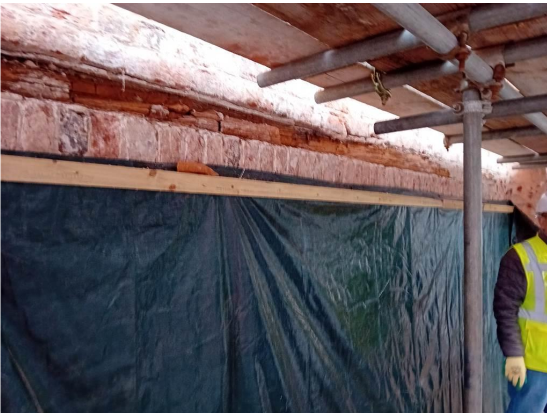
Photo 26: Merchants House: Wall plate no.1 built into the external walls.
