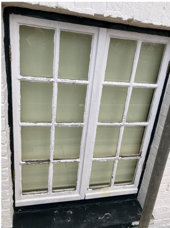
Photo 30: Victorian Sail Loft: Typical external windows W34 to W39.
